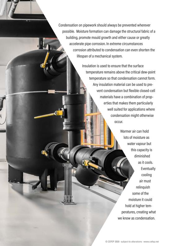
Any surface cooler than the surrounding air presents the potential for condensation but the risks are greater as the temperature decreases, making it a particular issue for refrigeration and air-conditioning pipes.
